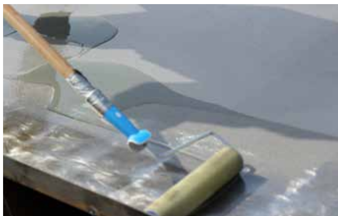
Figure 2: Priming the surface
