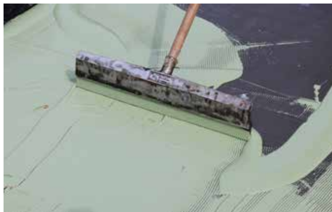
Figure 3: Binding the surface
