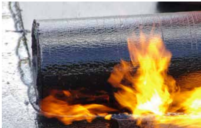
图3: 火焰加热Lucobridge®BIT
