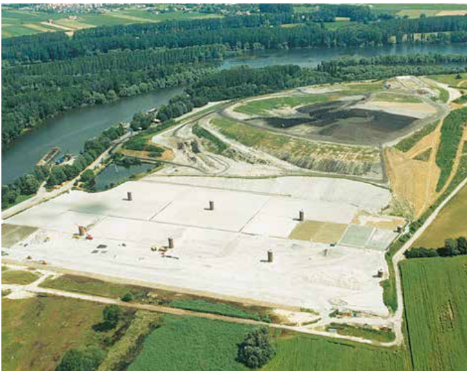
Sealing of landfills
