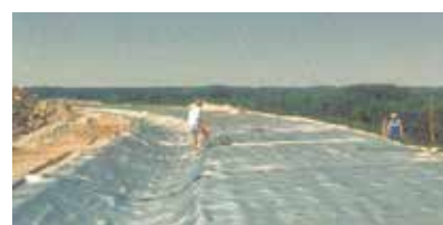
Landfill surface sealing
